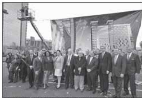
U/PAT members Vince Ramos and Kevin Bass, on boom, look over the gathering of downtown developers, politicians and labor leaders on the Marriott site.
